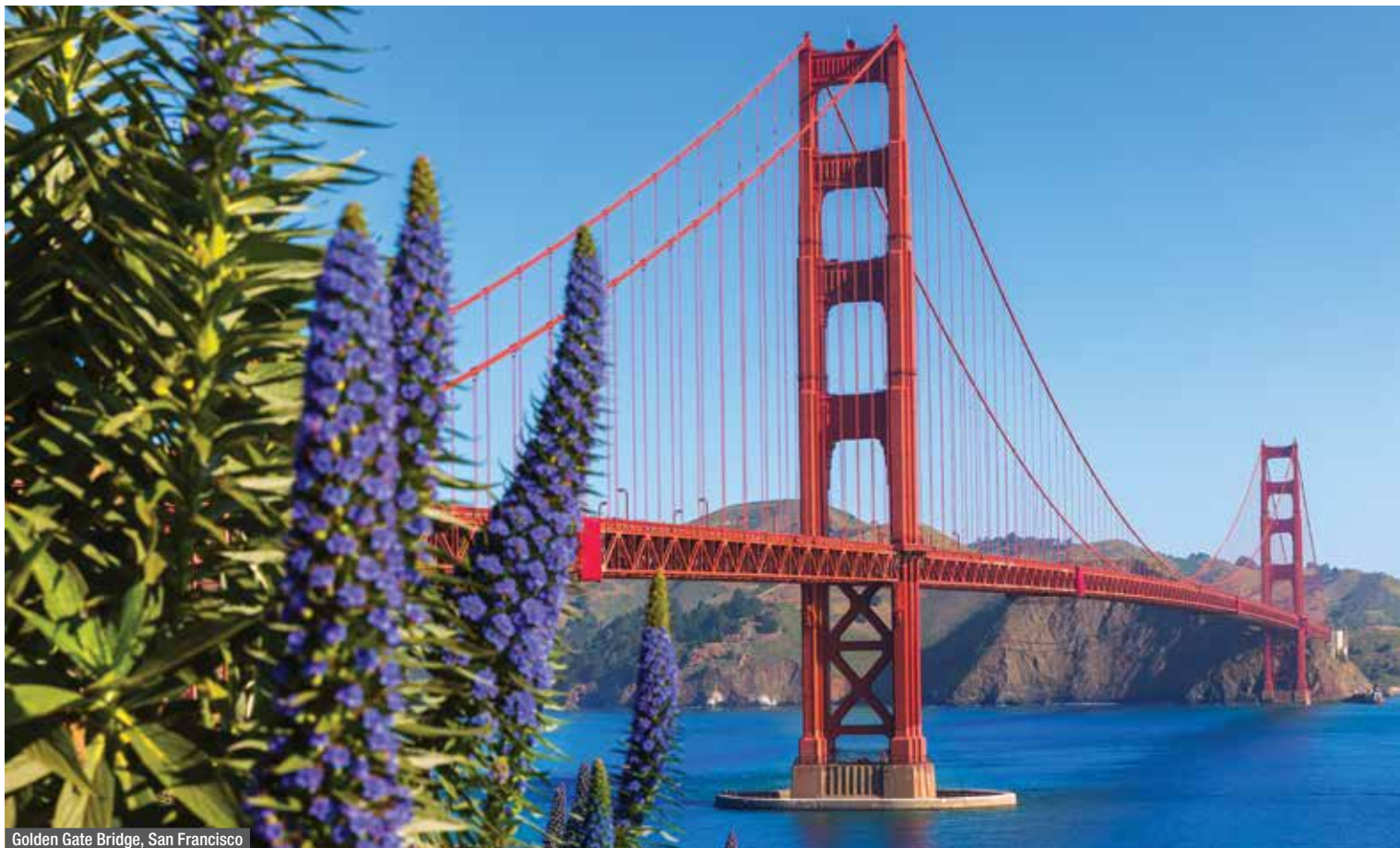
Golden Gate Bridge, San Francisco
